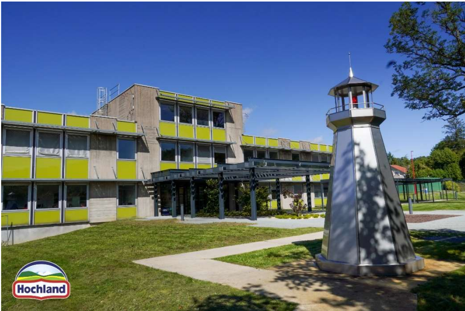
The plant in Dieue-sur-Meuse.
